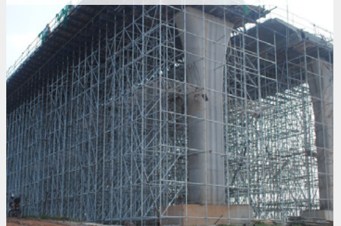
Quicklock scaffold for bridge construction
