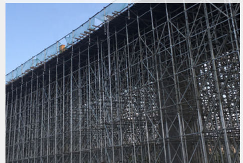
Quicklock scaffold for overpass construction
