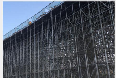
Quicklock scaffold for overpass construction
