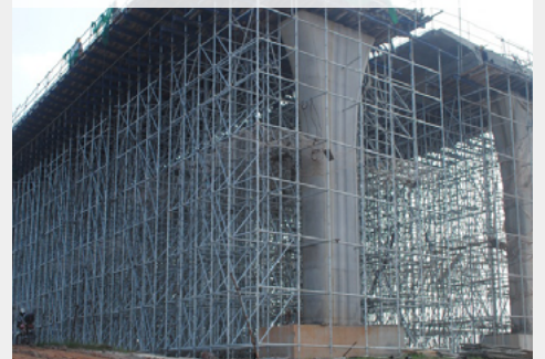
Quicklock scaffold for bridge construction
